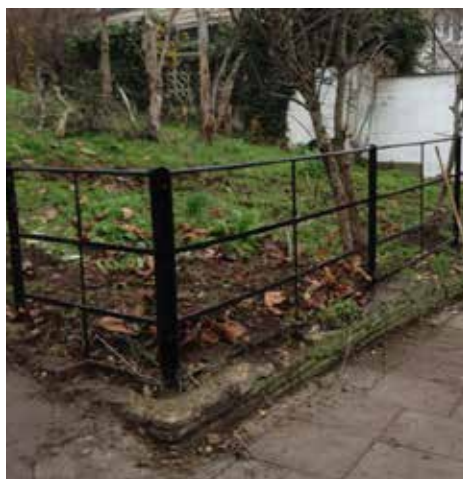
Newly installed estate railing
